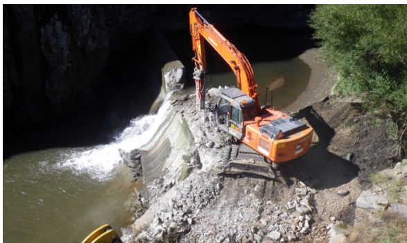
Odstránenie priehrady (hate) Gotera © Spanish Ministry of Agriculture and Fishing Food and Environment
